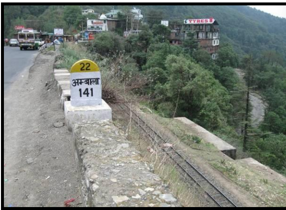
Road and Railway Line is Passing Side By Side Near Km 141+000 (Ex.)
