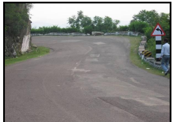
Blind Curve on existing Carriageway
