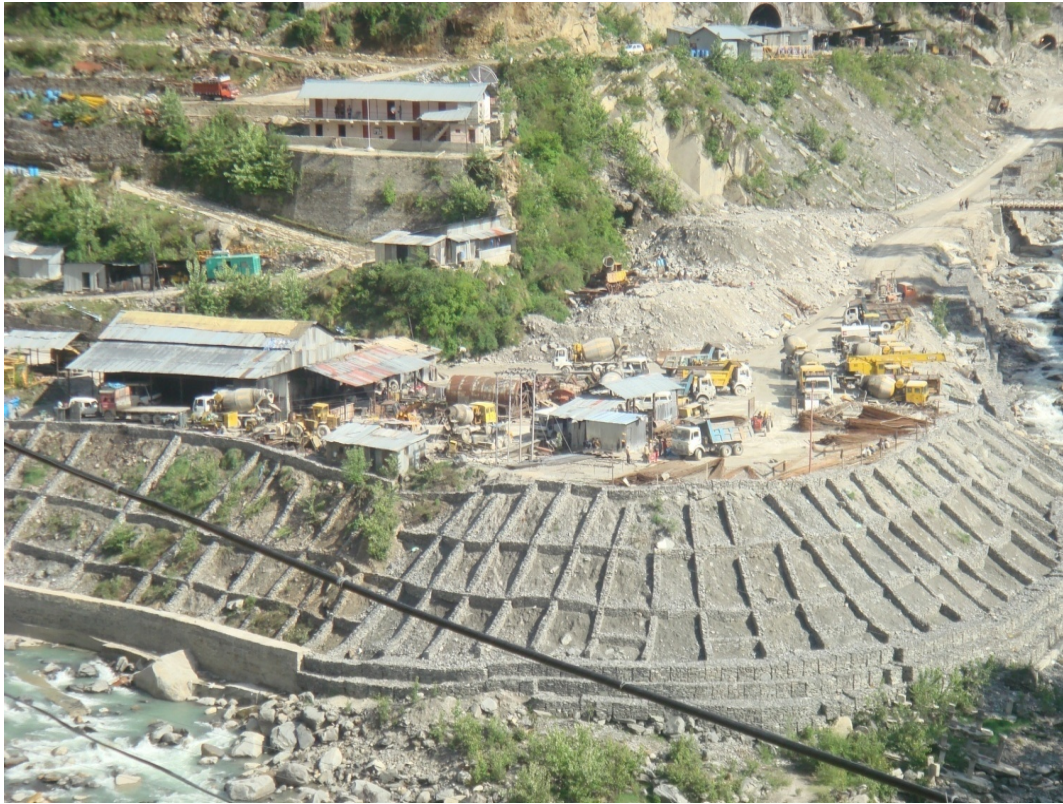
Figure – 4.2: Actual dumping site under restoration in a hydel project.
