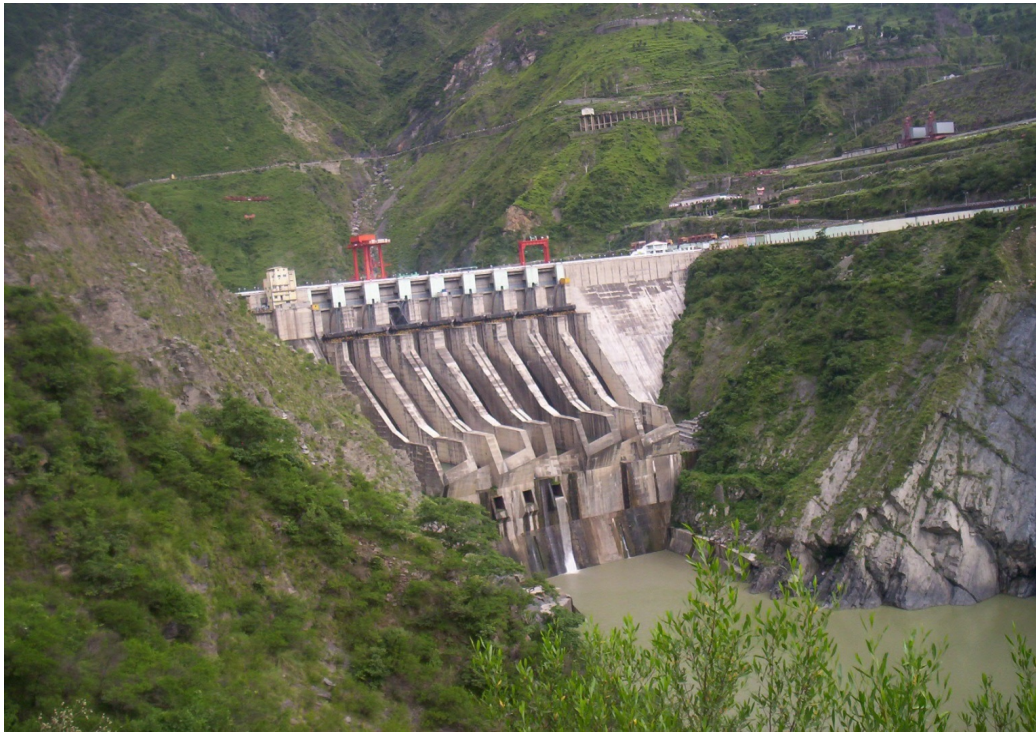
Figure – 4.3: Water release from the dam of hydel project.
