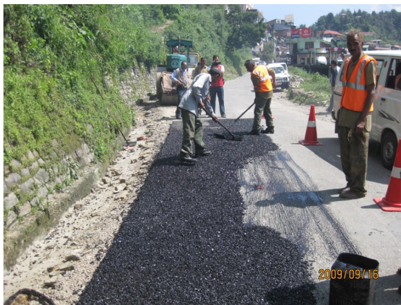
Figure -4.16 : Road Metalling using Plastic Mixed Bitumen
